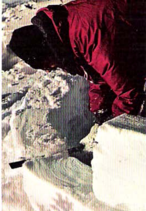
Each block must be sloped with a snowsaw or machete.
